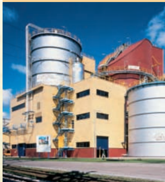
Flue gas desulphurisation plant in Elektrownia "Kozienice" S.A.
