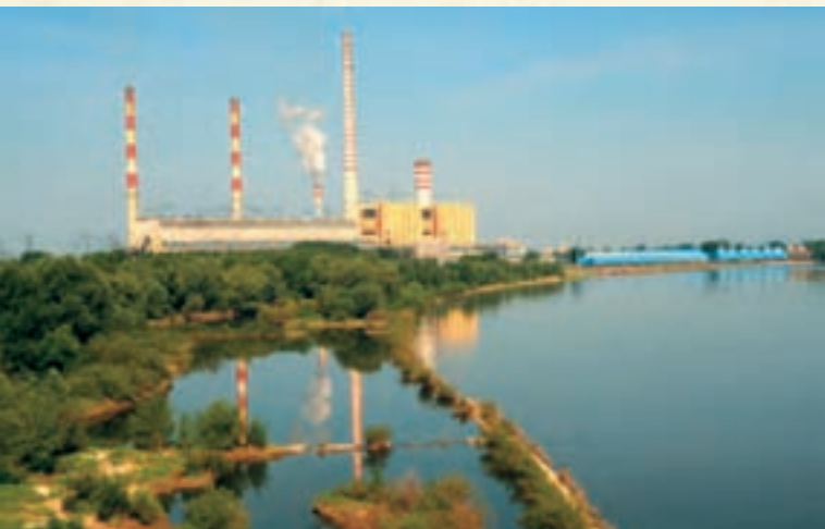
In Elektrownia "Kozienice" S.A. production of demineralized water to refill the boiler circulation of water and steam is carried out entirely with water from the Vistula river. In order to protect the river against thermal pollution, carried by spent cooling waters, effective fan cooling towers are being used.
