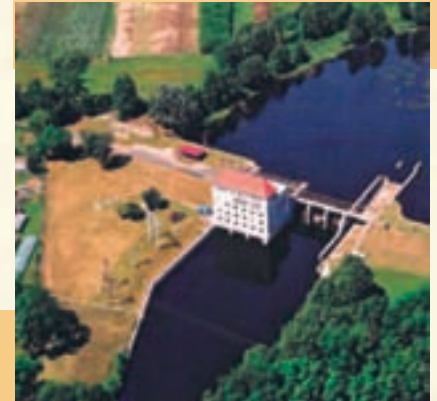
Hydropower plant in Dobrzyca.
